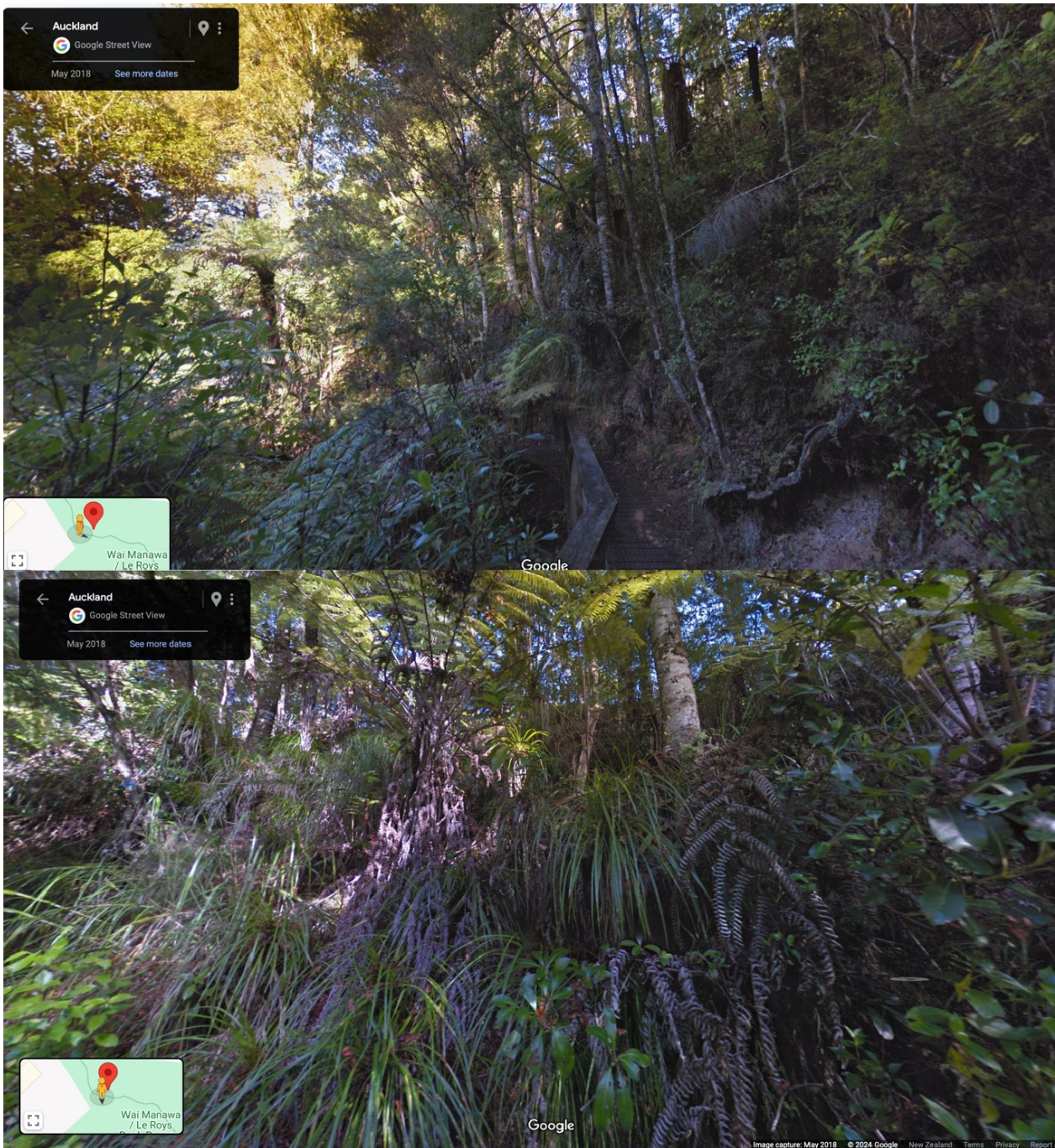
FIGURE 9: TRUE RIGHT BANK SLIP (SLIP 2) TOP (TOP) AND MID (BOTTOM) VIEW PRIOR TO THE CYCLONE
