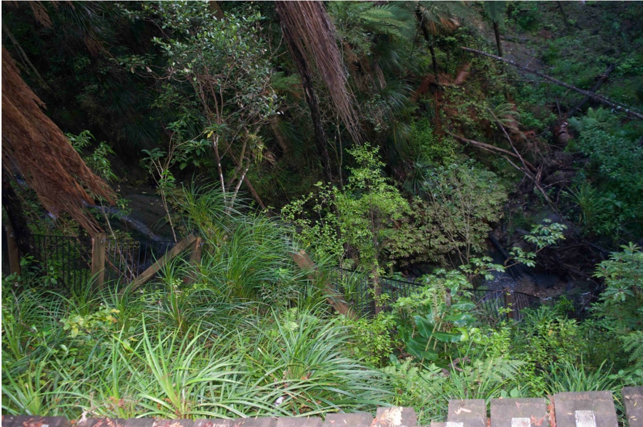
FIGURE 21: HANGING INFRASTRUCTURE IS HAZARDOUS
