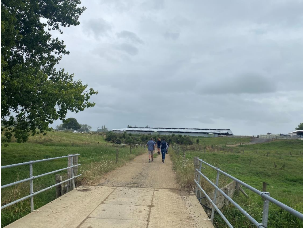
Figure 4: Bridge over Piako river near Kereone
