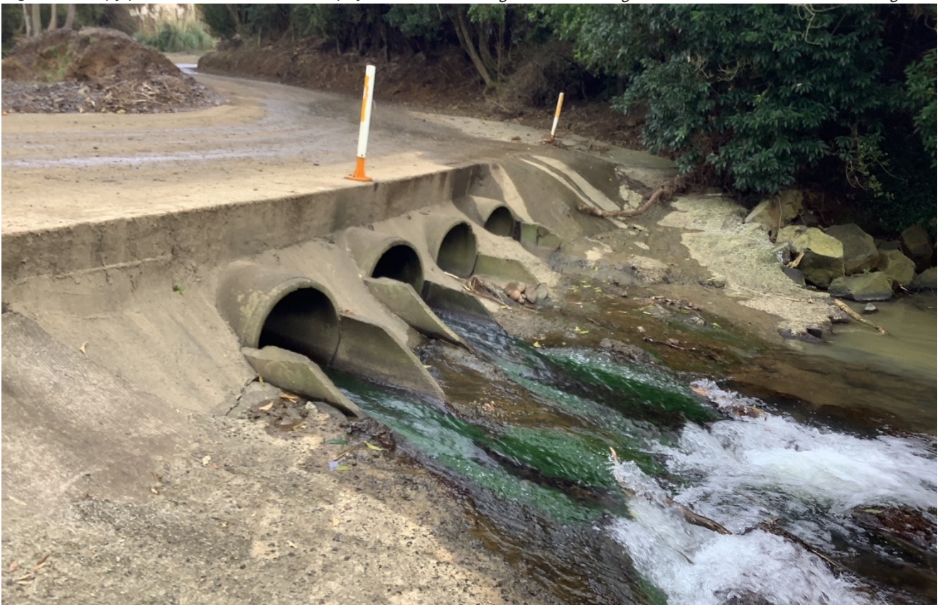
Figure 10. Ford and culverts at Makaewa Road.
