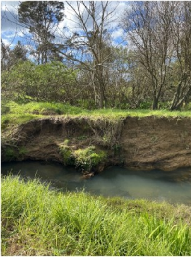
Figure 5. Erosion scars along TLB.
