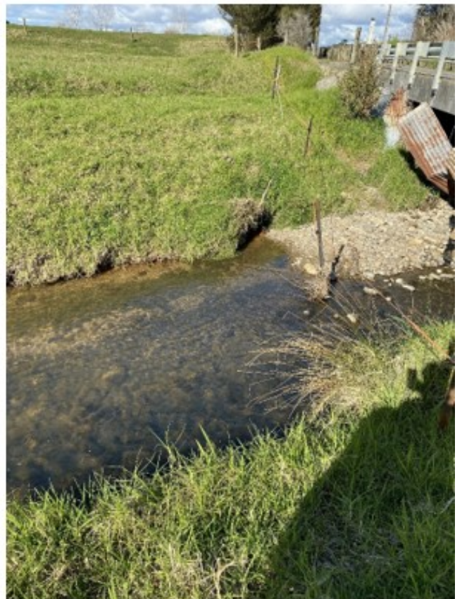
Figure 9. Green algae on streambed at Toft Road Bridge.
