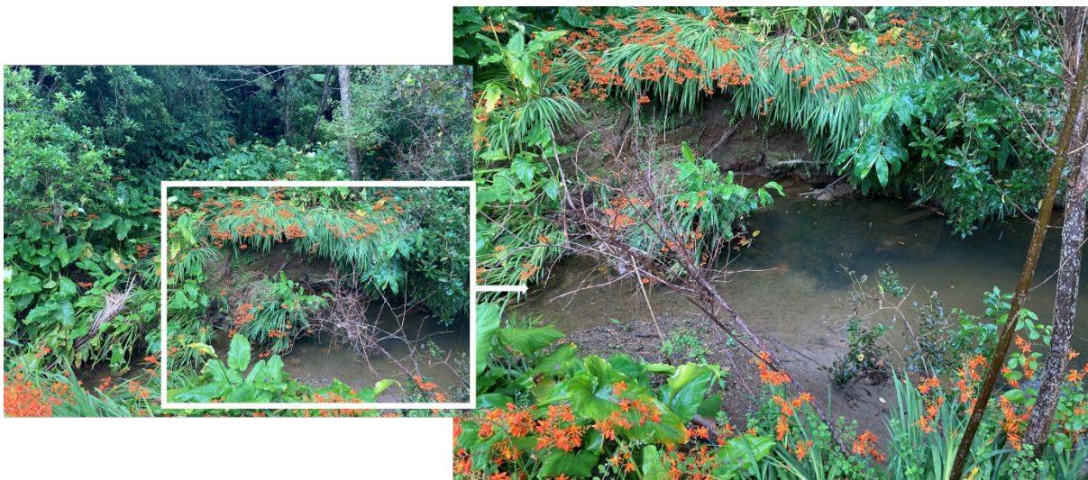
Figure 5. Bank erosion and bed scour at swimming hole
